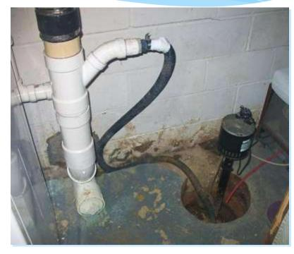
This photograph shows an illegal connection of a basement sump pump to the sanitary sewer line. In the Village of Cazenovia, such connections are illegal.
