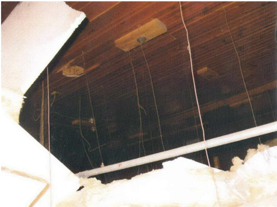
Dead Space above dropped ceiling
